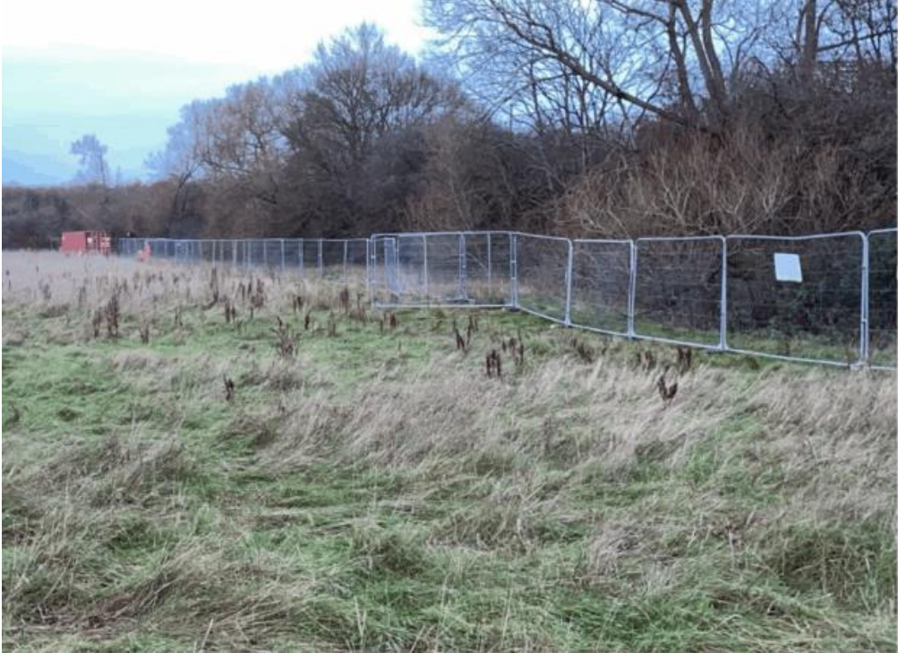
Securing of the Site November 2025
